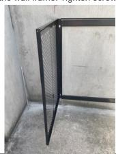
3. Slide the top panel into the guides on the sides.
